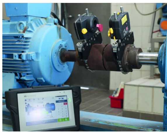
Optalign Touch aligning the shaft of a pump
