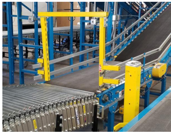
Install & maintenance of conveyor belt system
