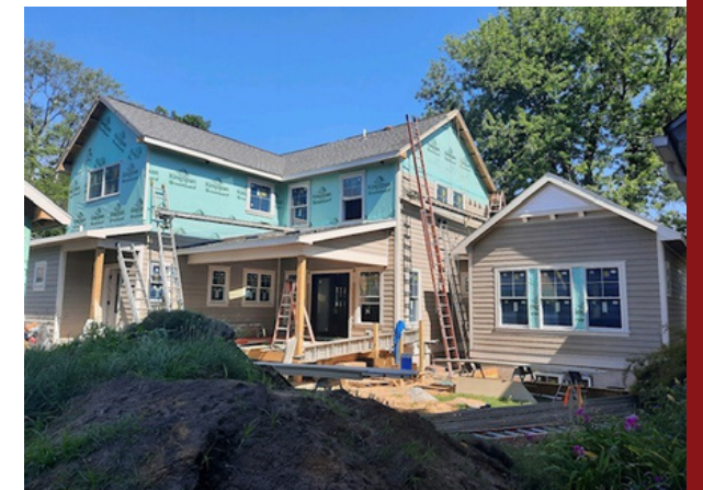
New home construction
