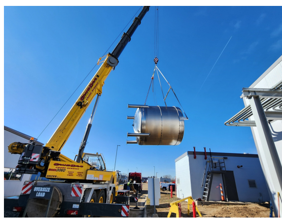
Crane pick for Tank Install
