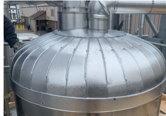
Vessel Head Replacement
